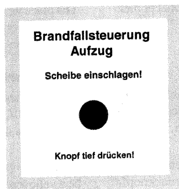
Fig. 5. Sample of a push button call point for the manual triggering of the fire control system
